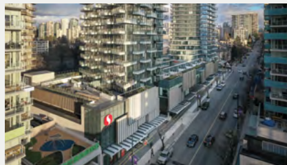
Davie Street Vancouver, British Columbia Major development
